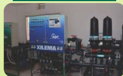
Automatic Fertigation and Filtration Unit
